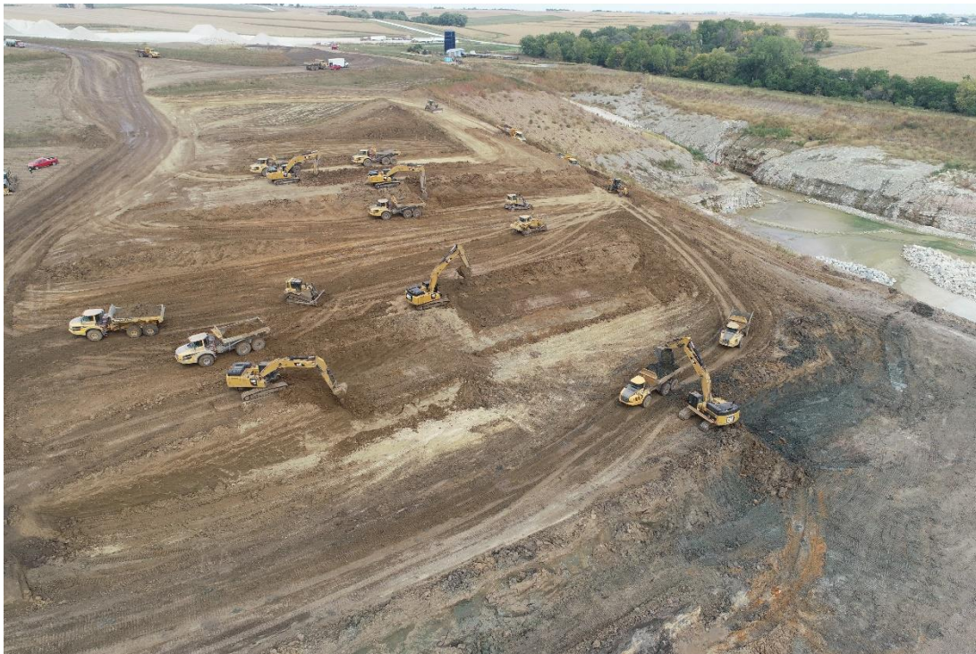
Stripping of a quarry location
